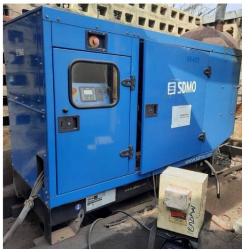
Diesel generator that provides power supply on the Customer's facility (GSM mast)
