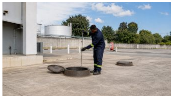
Fuel level measurement with a dipstick
